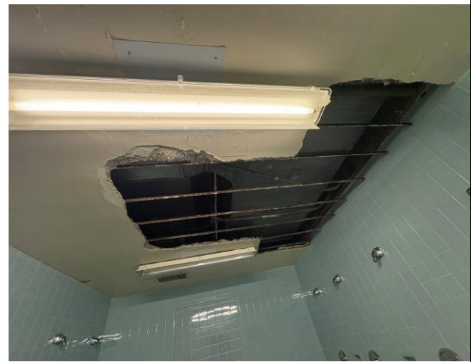
Figure 4: General view opening present on plaster ceiling within Girl's Changeroom.
