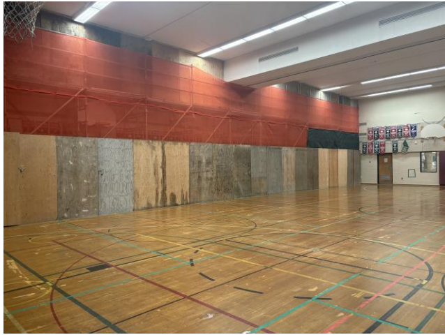
Figure 1: View within the Gym with plywood hoarding and debris netting on east side.
