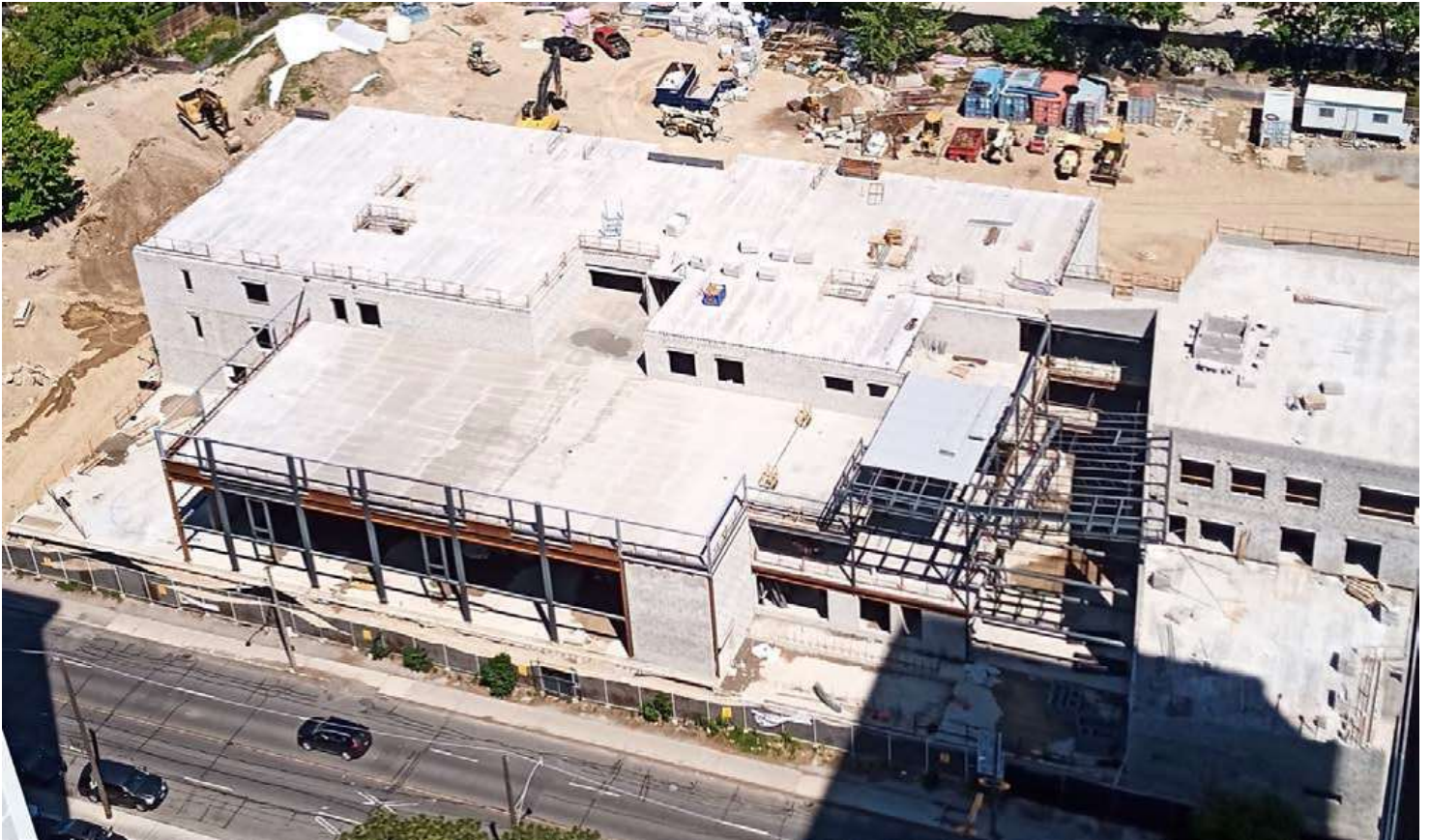
OVERVIEW OF CONSTRUCTION – June 2020
