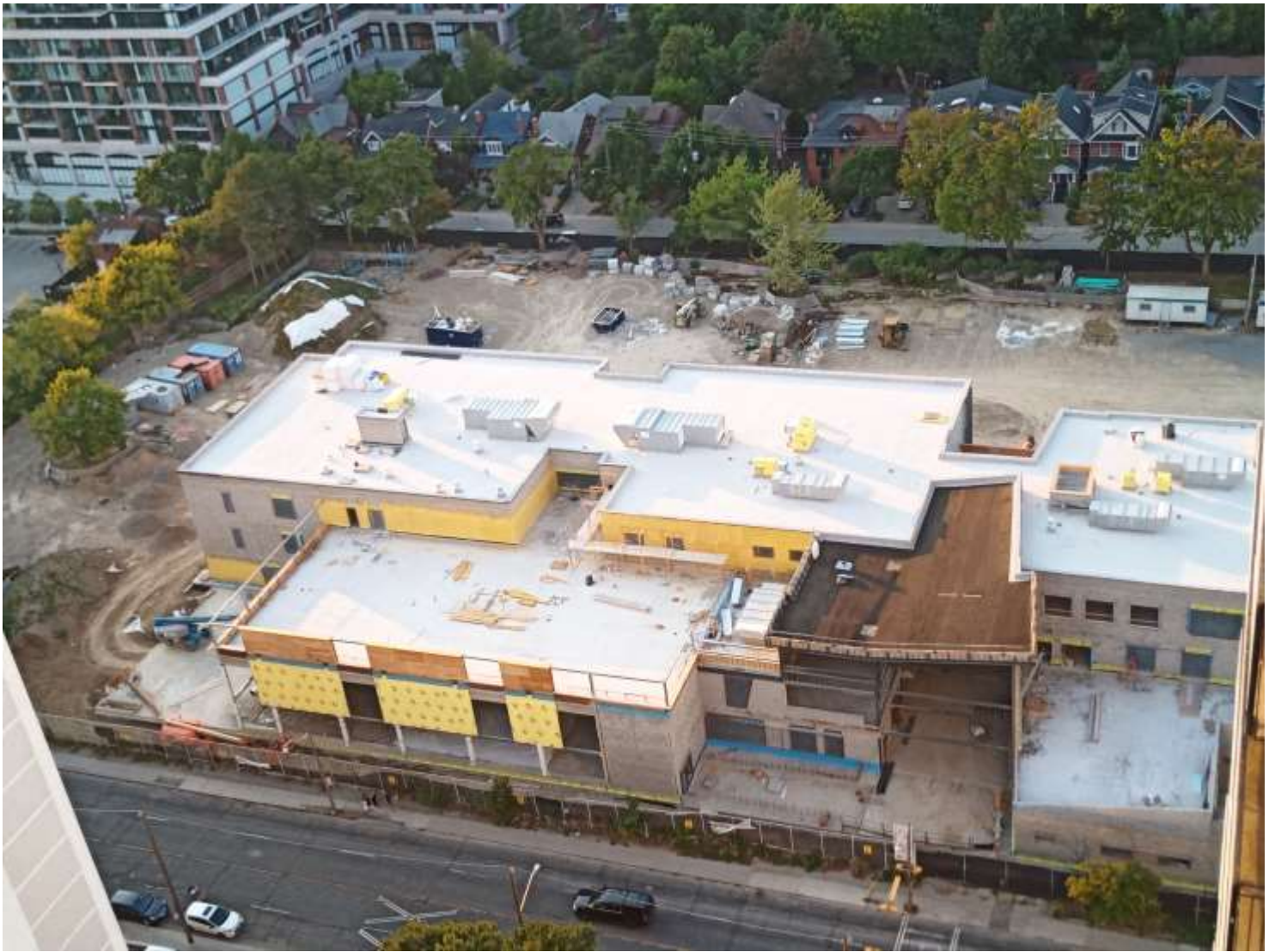
OVERVIEW OF CONSTRUCTION – August 2020
