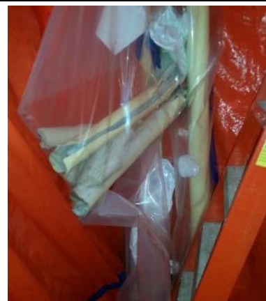
Photo 6: After Removal, Inside Glove Bag
