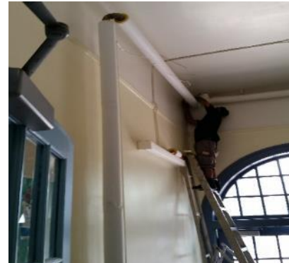
Photo 9: Pipes Reinsulated with New Fibreglass Insulation
