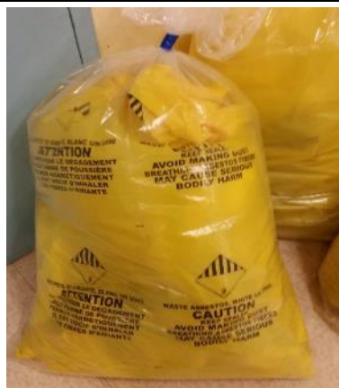
Photo 5: Asbestos Waste Double Bagged
