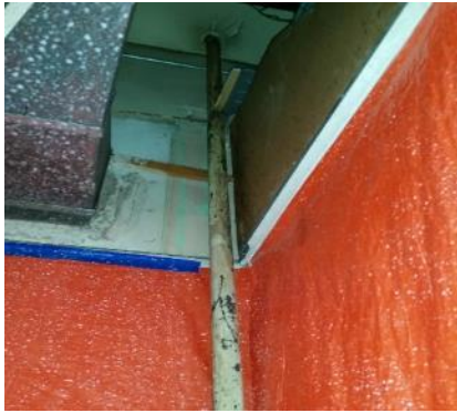
Photo 7: Pipes After Removing Glove Bags
