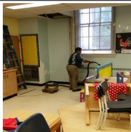
Photo 10: Final Mopping and Vacuuming
