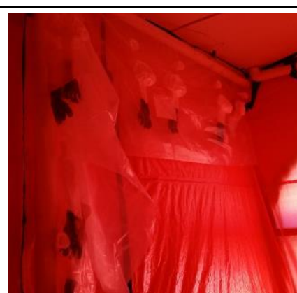
Photo 3: Glove Bag Enclosure Setup Inside the Full Enclosure
