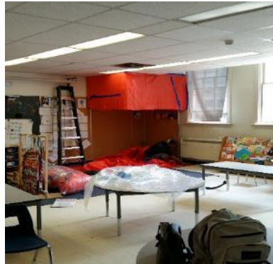
Photo 8: Tear Down of Type 2 Full Enclosure
