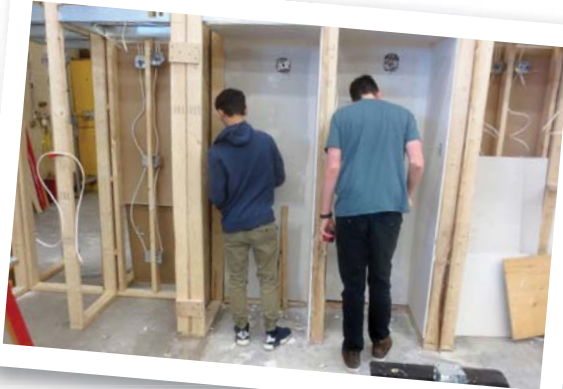
Students measuring counter top height for support rails
