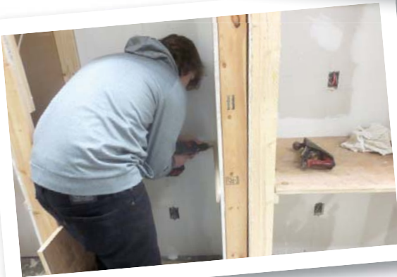
Student installing the cleats for a counter top in grade 11 Construction Engineering
