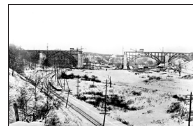
Building the Prince Edward Viaduct over the Don Valley, 1918
