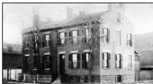
Typical Row Houses of the 1860s (on Sherbourne Street)
