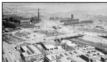
Building the new Waterfront circa 1929
