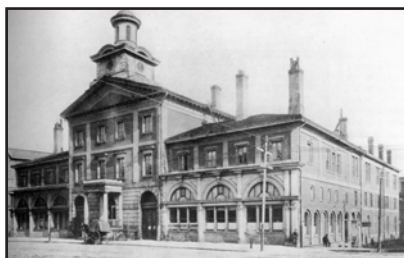
Toronto's City Hall (south west corner of Jarvis and Front) circa 1867
