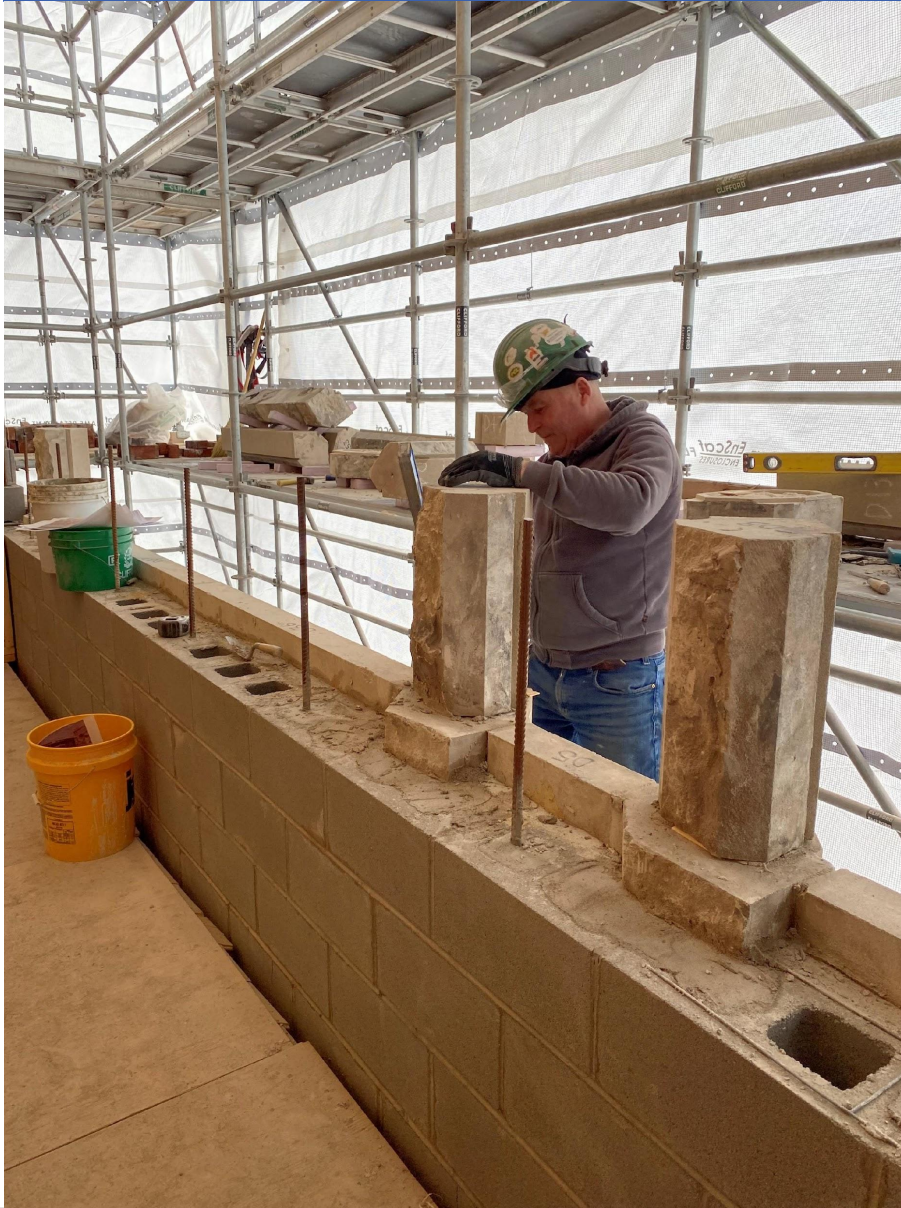
Restoration of the 1929 front façade east bay.
